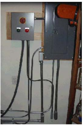
Here is the user interface for the phase converter. It is mounted next to the garage distribution panel. I have the two pushbuttons for start and stop, plus a disconnect switch for control power.
